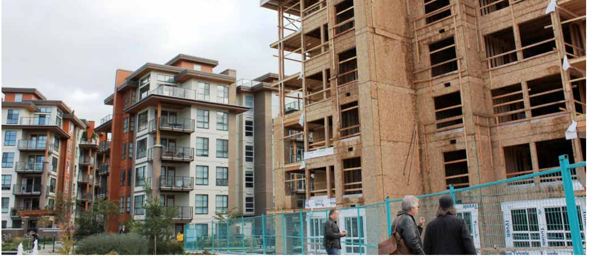
Mid-rise wood-frame buildings in Vancouver, B.C. are bringing quality, safe and new housing types to the city including condominiums and rental.
