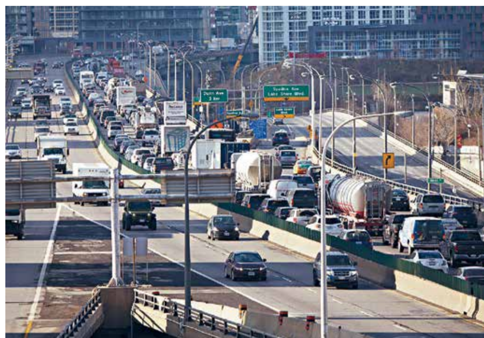
Roads and highways — part of our city’s infrastructure — are fundamental to our daily lives, support growth and are essential to the economic prosperity of our city, region and nation. FILE PHOTO/TORONTO STAR
